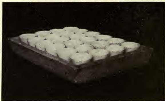
FIG. 21. — Clay dish holding 24 annealing cups.
